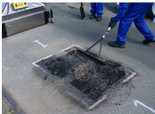
Reworking of in situ surfacing material
