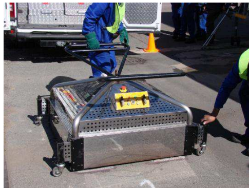
Positioning of infrared heater over surface area to be repaired
