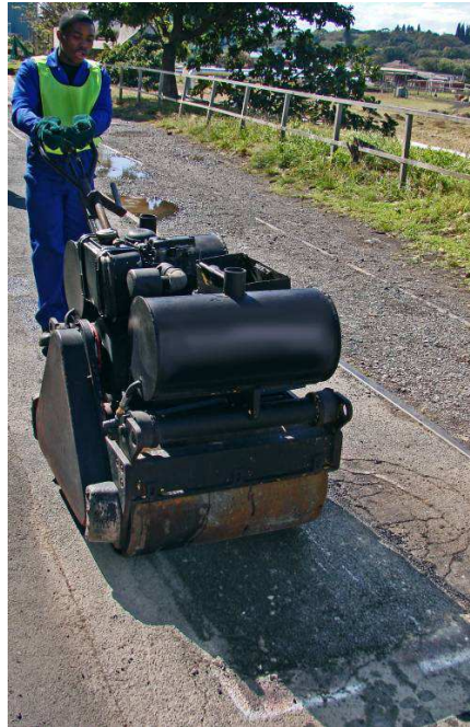
Rolling being completed
