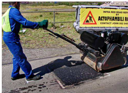
Compacting of repaired surfacing
