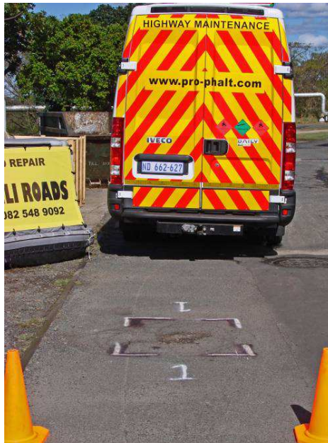
The Pro-Phalt van being backed up to the damaged road surface
