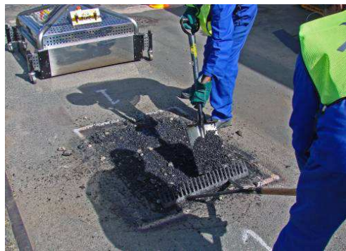
New material being added and mixed with in situ material
