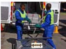
The portable infrared heater is positioned over the defect and heats the surface area to approximately 200°.
